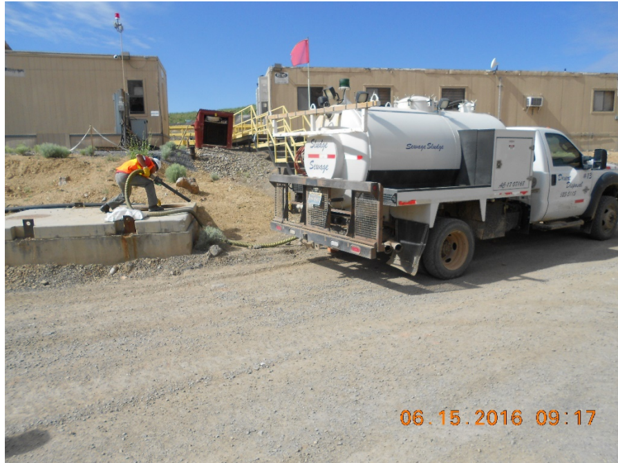
Fig. 4 - Pumping a Vault Holding Tank
